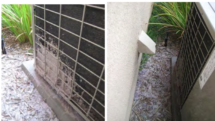
Figure 11- 35 : Noncompliant Condensing Unit Clearance from Dryer Vents
