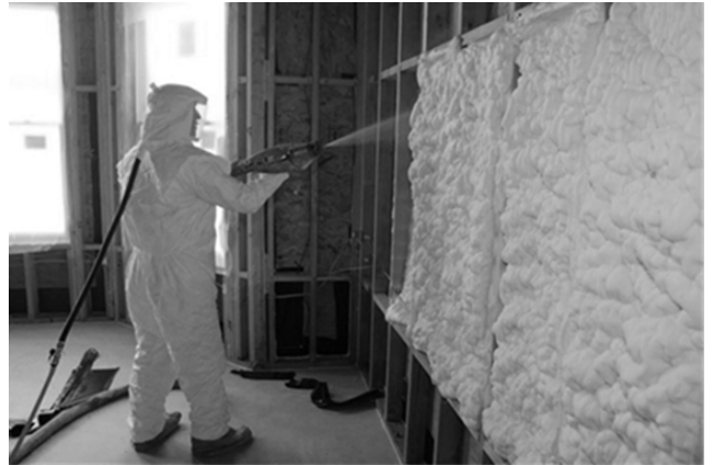
Figure 3-17: Open-Cell SPF Installed in Wall Cavity
