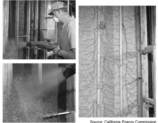
Figure 3-15: Cellulose-Insulated Wall
