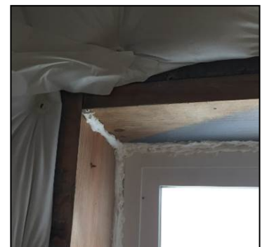
Figure 3-10: Air Sealing
