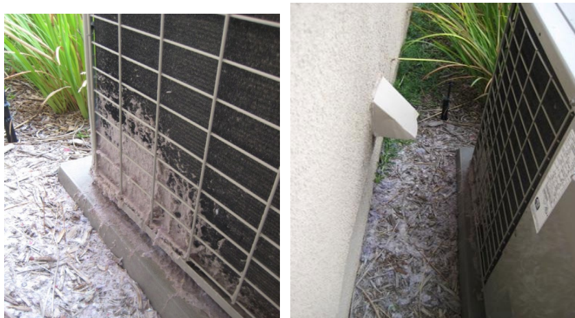
Figure 4-2: Noncompliant Condensing Unit Clearance From Dryer Vents
