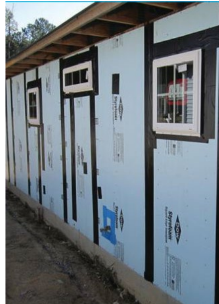
Figure 3-19: Properly Installed Rigid Insulation With Sealant Tape
