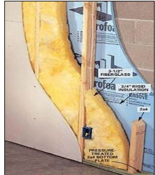
Figure 3-29: Masonry Wall With Furring Details
