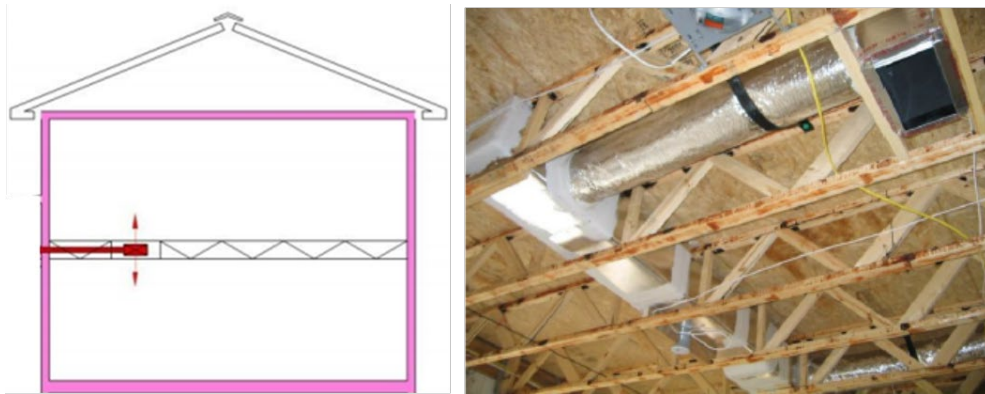
Figure 4-13: Open Web Floor Truss Example
