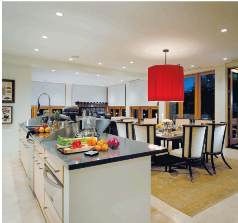
Figure 6-1 Recessed Downlight Luminaires in Ceiling
