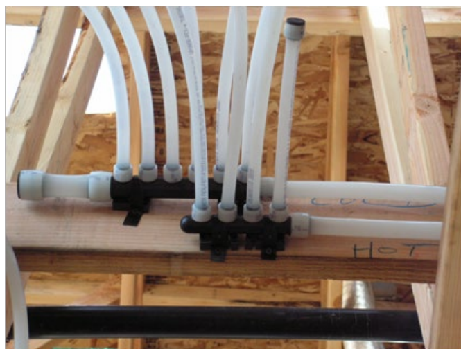
Figure 5-9: Mini-manifold Configuration
