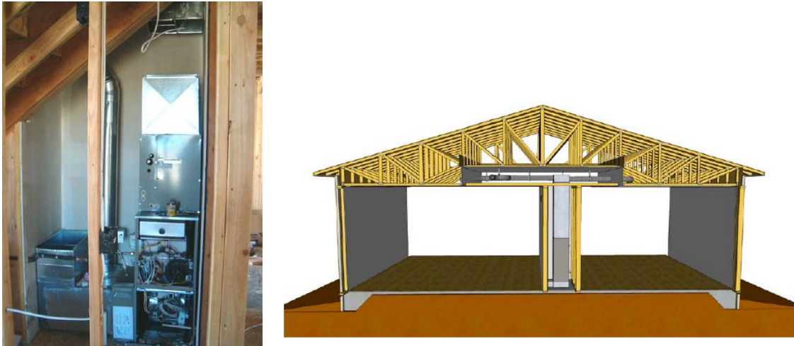
Figure 4-14: Mechanical Closet Placement Example
