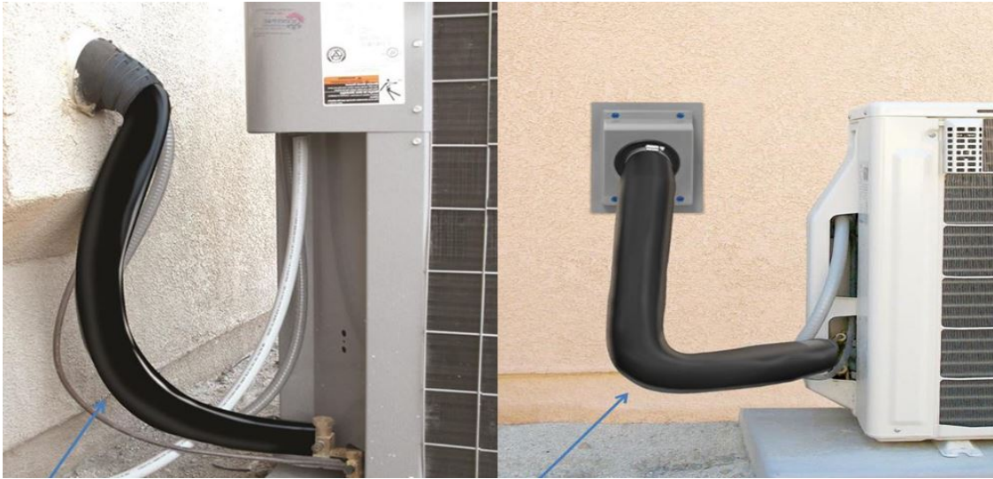
Figure 4-1: Refrigerant Line Insulation
