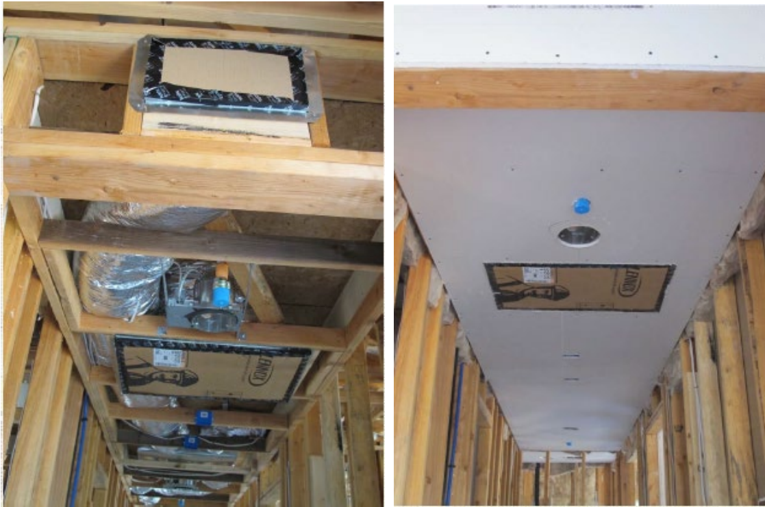
Figure 4-11: Ducts Routed Through a Dropped Ceiling
