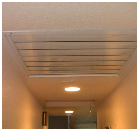
Figure 4-38: Whole-House Fan With Barometric Damper
