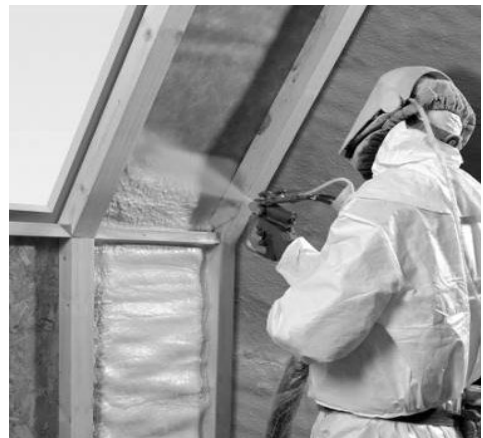
Figure 3-18: Closed-Cell SPF Installation in a Wall Cavity
