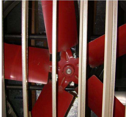
Figure 4-39: Open Barometric Damper With Fan Above
