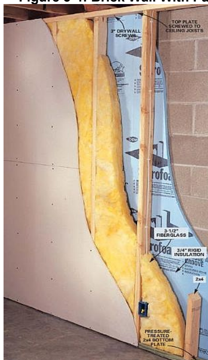
Figure 3-4: Brick Wall With Furring Details
