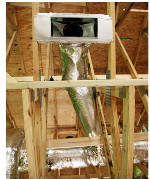
Ductwork in Attic
