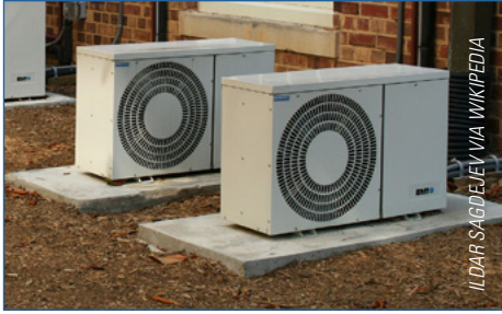
Ductless Mini Split System, outside unit
