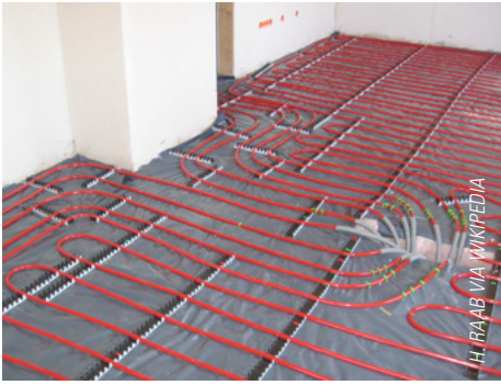
Raidant Hydronic System
