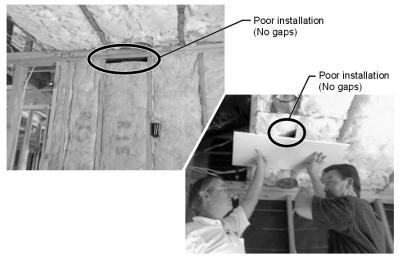
Figure 3-46: Examples of Poor Quality Insulation Installation
