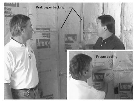
Figure 3-13: Typical Kraft Faced Vapor Retarder Facing
