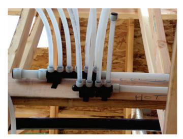
Figure 5-8: Mini-manifold Configuration
