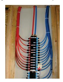
Figure 5-9: Central Manifold System
