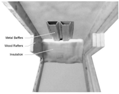
Figure 3-29: Baffles at the Eave in Attics
