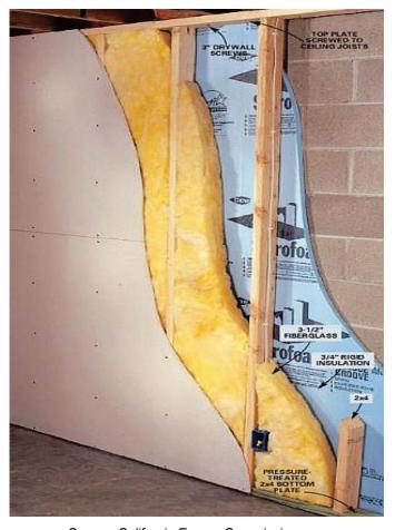
Figure 3-32: Masonry Wall With Furring Details
