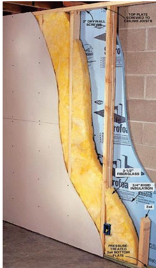
Figure 3-4: Brick Wall With Furring Details
