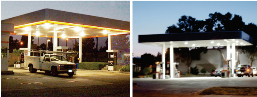
Figure 6-4: Service Station Hardscape Areas
